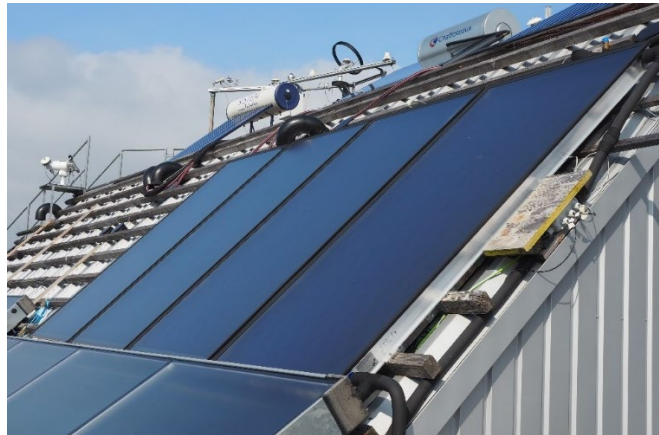
Figure 52: The four collectors of the demonstrator DBS mounted on the roof in parallel.
