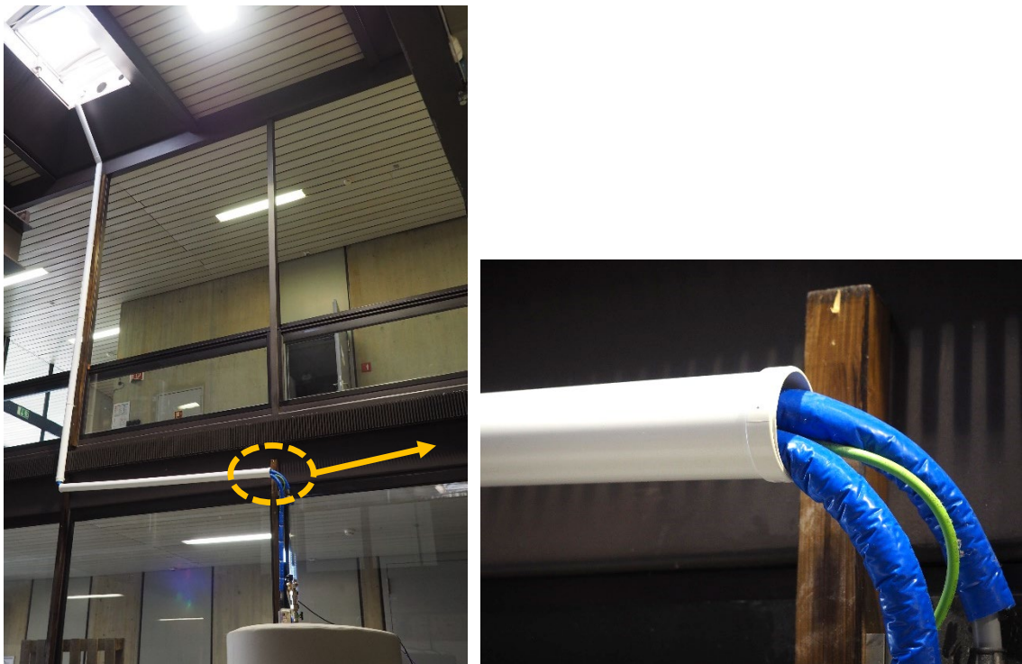
Figure 54: Solar loop, left: section inside the building, right: detail with opening of the waterspout pipe with the two pre-insulated solar pipes (in blue) and an electric cable of the monitoring sensors.
